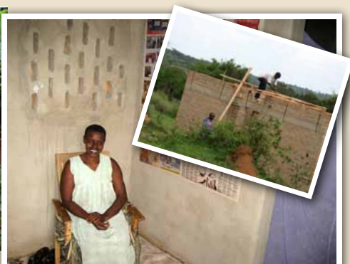
Substantial houses like this one give families secure protection against the elements
